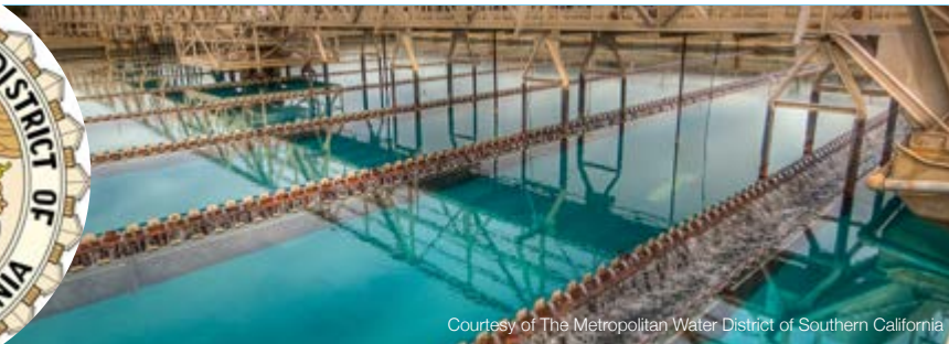
Courtesy of The Metropolitan Water District of Southern California
